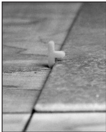
Fig. 11 - Use spacers with one leg removed.
