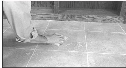
Fig. 21 - Use a 3M white, nylon pad to loosen grout residue.
