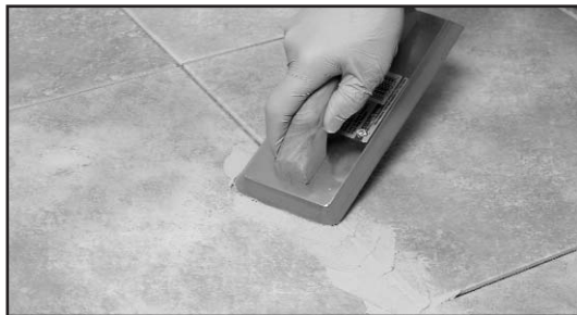
Fig. 19 - Pack the grout into the joints.
