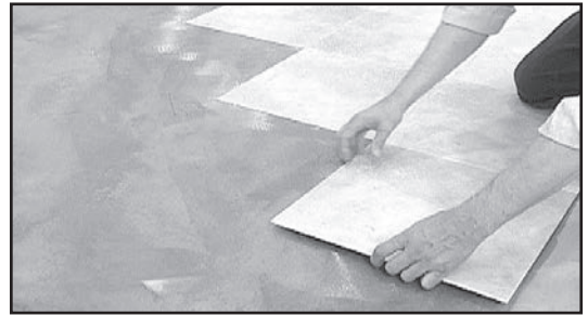
Fig. 14 - Install ungrouted floors following a stair-step pattern.
