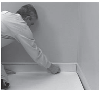
Fig. 2. Cut leaving 1/8" to 1/4" space at perimeter.
