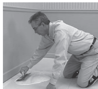
Fig. 4. Apply adhesive and install product.
