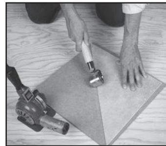
Fig. 18 - Roll the cut edge to form a slight radius.
