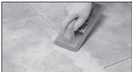
Fig. 19 - Pack the grout into the joints.
